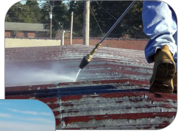
Power washing roof after RustArrestor™ application.
