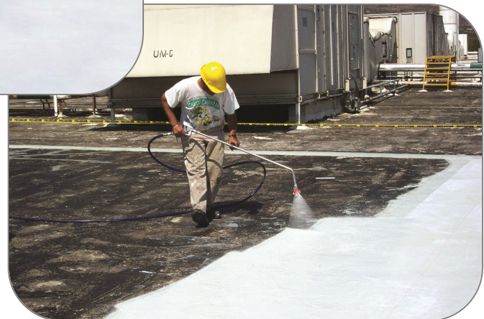
Topps Seal® Base Coat applied by spray.
