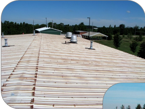
Metal roof prior to coating is leaky and rusted.
