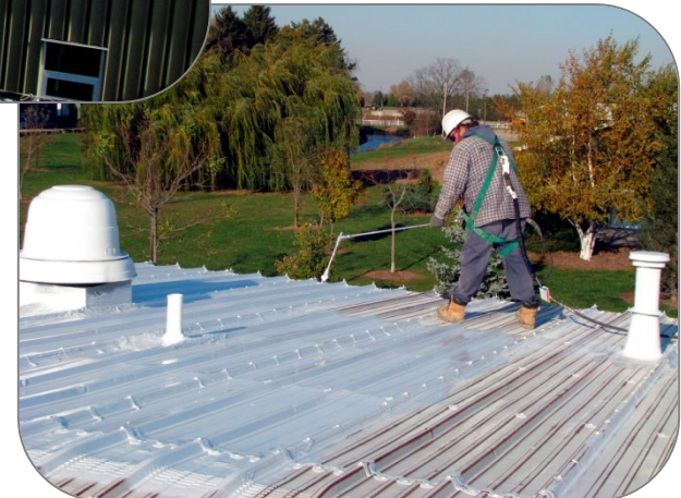
Spraying Topps Seal® Base Coat.
