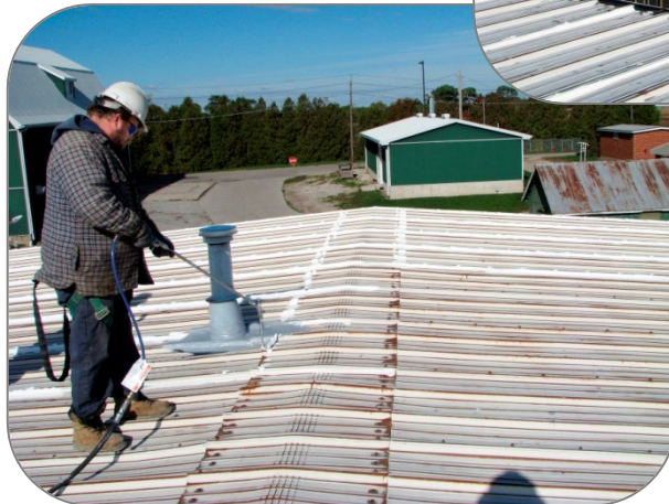
Seams sealed with RivetGuard™.
