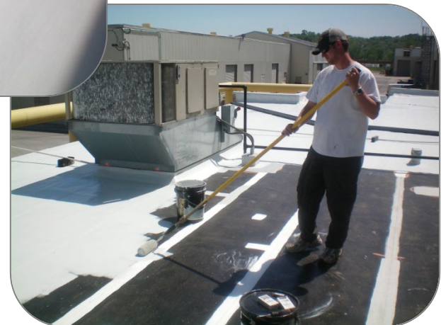
Topps Seal® Base Coat applied by roller.
