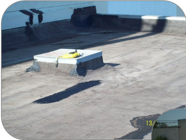
Felt roof prior to coating.
